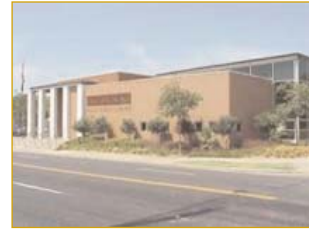
Successful joint venture between private supermarket developer and public library
